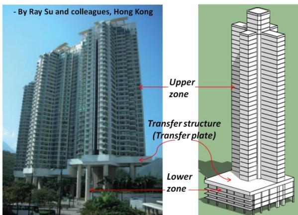
Fig. 1: Transfer-plate high-rise building (TPHRB)
